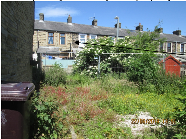
Rear elevations of houses on Gordon Street
